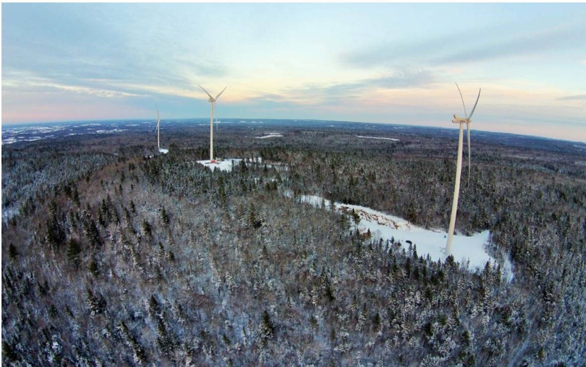
The W.E.B wind turbines in Nova Scotia survived the hurricane undamaged.
