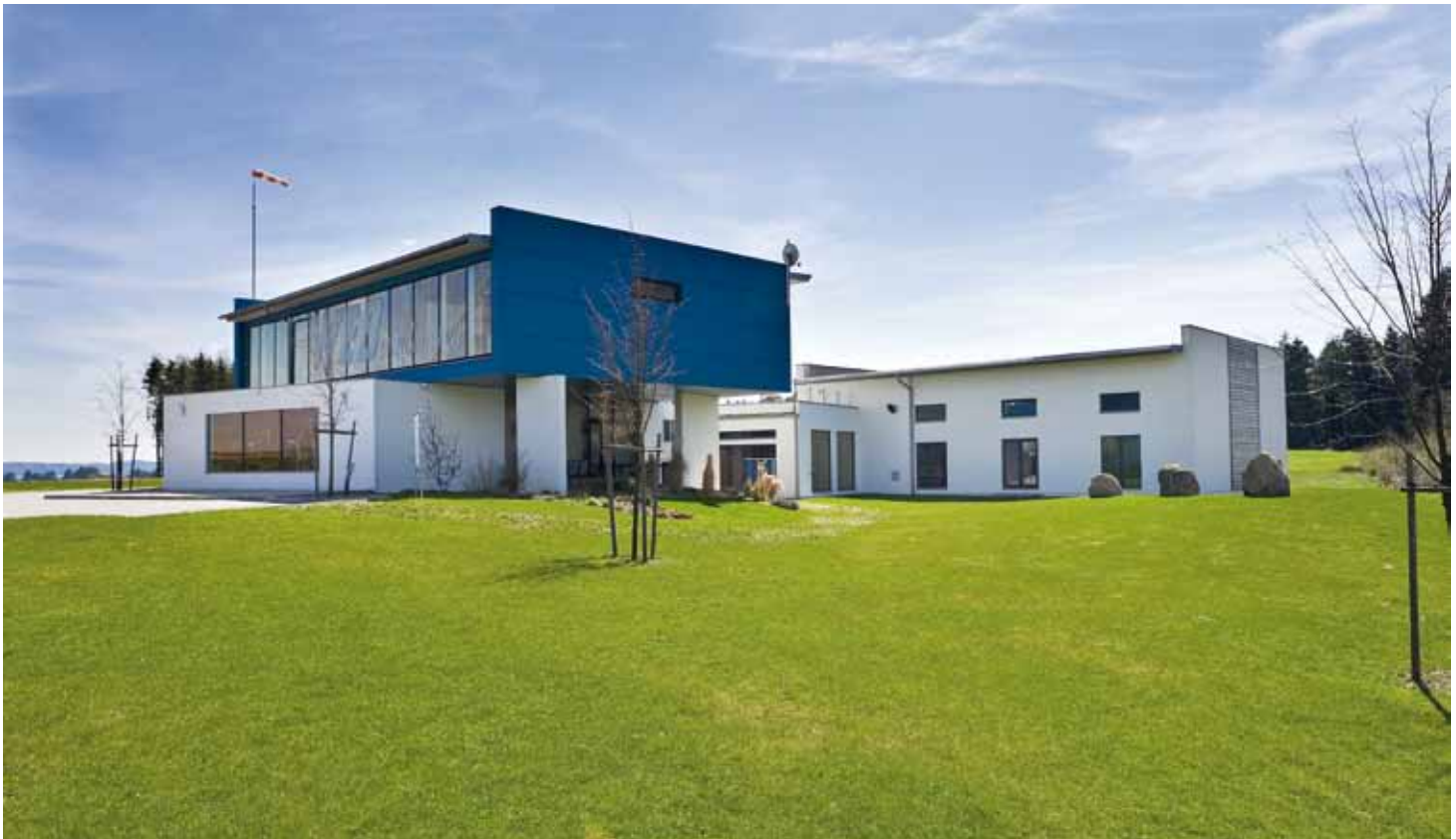
Corporate headquarters in Pfaffenschlag/Lower Austria
