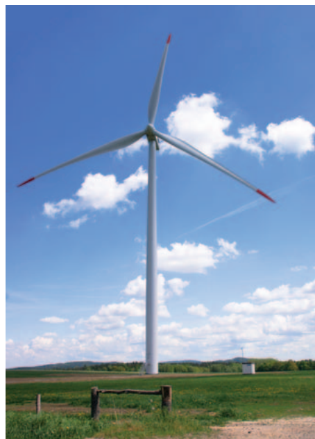
The first W.E.B plant with 100 m rotor diameter
