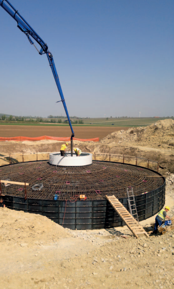
Work on the building site in Höflein.
